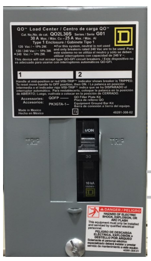
240V to AC or Heat Pump Compressor
